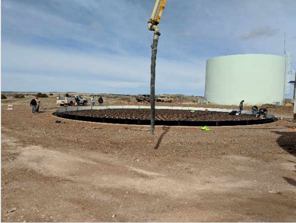
Before and after pictures of the 1 million gallon storage tank replacement at the Rolling Hills well site
