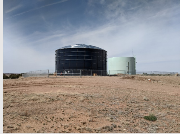
Before and after pictures of the 1 million gallon storage tank replacement at the Rolling Hills well site
